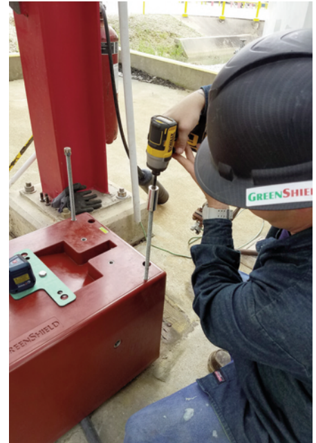
Threaded leveling screws with PoxyVials™
